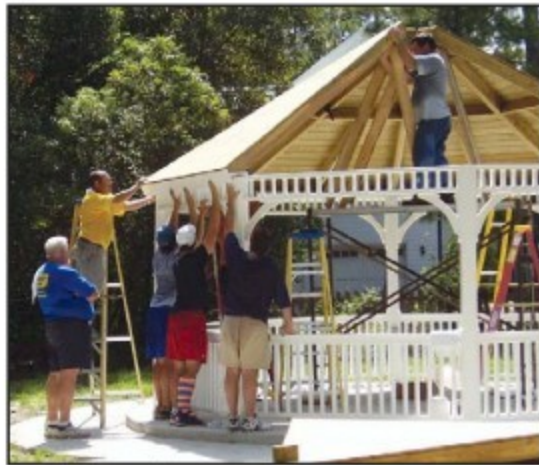
Raising the roof!
